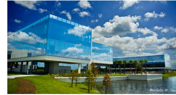
DARDEN RESTAURANTS CORPORATE HEADQUARTERS Orlando, Florida
